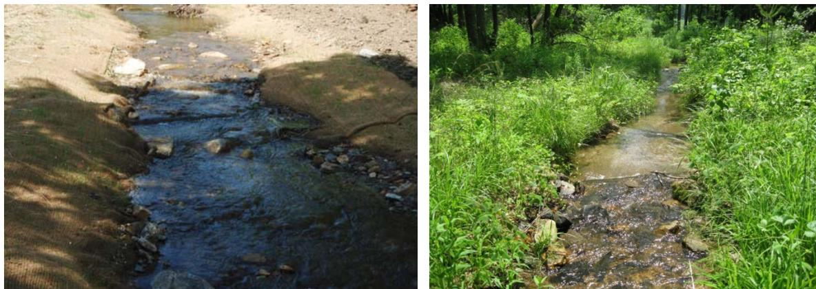
12 **Figure 9: Examples of Log/Rock Constructed Riffle**
